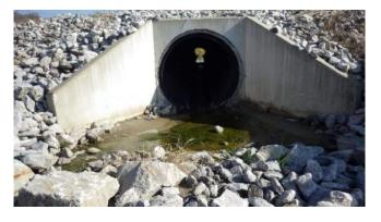
The southern of two final grade surface/storm water channel culverts passing beneath the access road to the temporary construction office trailers. A slight bow was observed in the crown.
